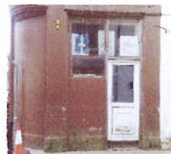
12 Cross St unoccupied more than five years
