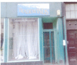
11 Main St unused for retail eighteen months
