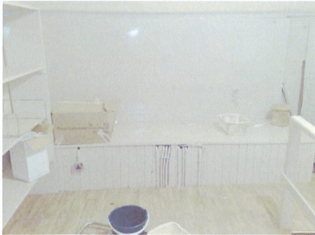
Upper level showing services bulkhead
