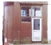
12 Cross St unoccupied more than five years
